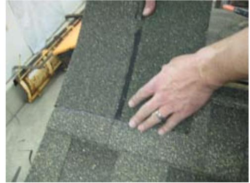
Install the first ridge cap. Make sure it is at the chalk line as shown, and secure with 1 1/4" roofing nails.
