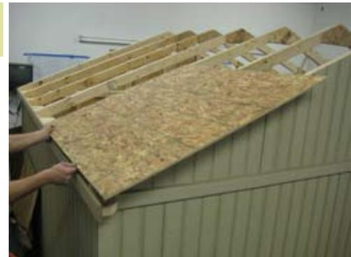
Next install roof sheathing. See roof layout for proper roof sheathing placing.
