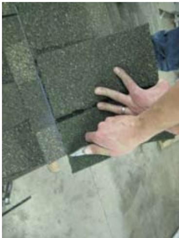
Second to last ridge cap is being installed. Cut off whatever overhangs over the roof.
