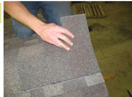
Next cut ridge cap to complete the roof.
