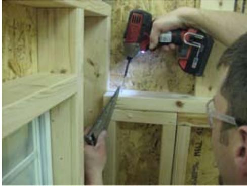
Make sure bottom plate of gable and top plate of end wall are flush on the inside.
