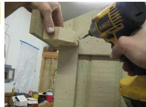
secure rake block with 2 1/2" zinc screw.
