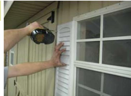
Make sure shutter is evenly spaced up and down with window and secure with white head screws provided for shutters.
