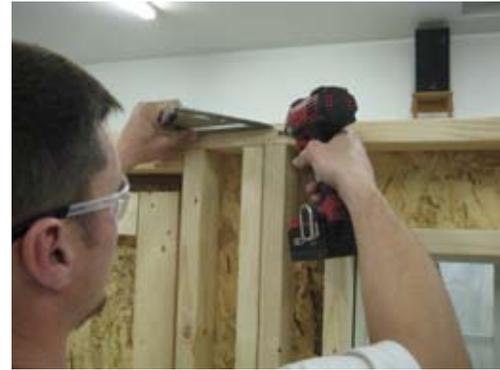
Once bottom is secured, make sure top end is flush as shown and secure with 2 1/2" screws.
