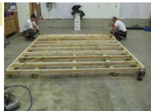
Once the 2x4's are secure on sides and both ends, measure from corner to corner to square up floor.
