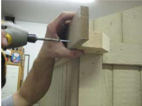
Insert 1 1/4" zinc screw from fascia trim into rake block as shown.
