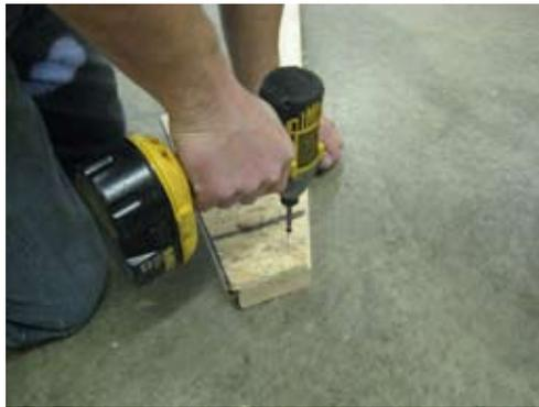
Secure on truss and heel with 1 1/4" zinc screws.
