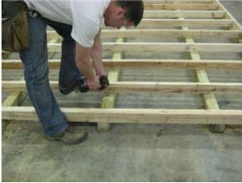
Once floor is square, secure each joist by using a 2 1/2" screw as shown.
