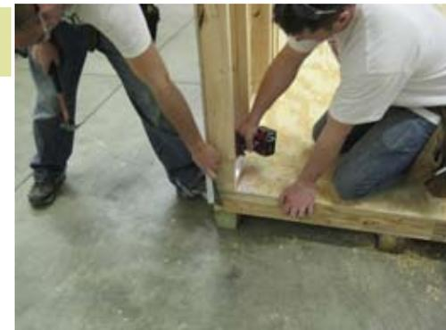
Make sure wall is flush as shown. Secure wall to floor with 2 1/2" screws.
