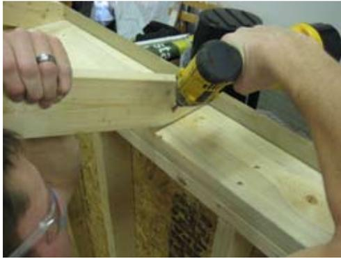
Insert screw on angle as shown to secure truss.
