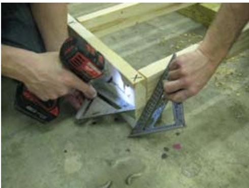
Next make sure joist and rim are flush with 4x4 runner and secure with 2 1/2" screws.
