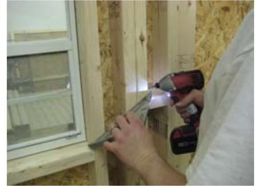
Secure wall splices with 2 1/2" screws.
