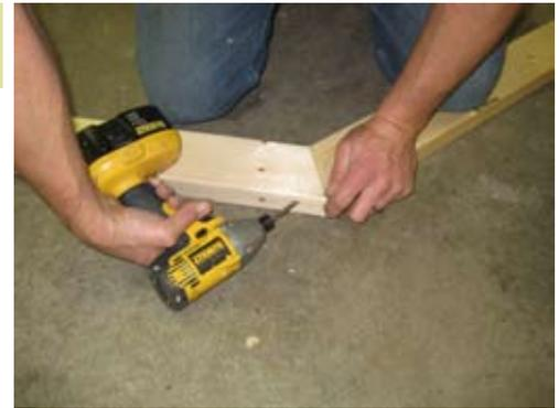
Make sure peaks line up and secure with 2 1/2" zinc screws as shown.
