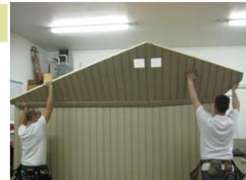
Lift gables to set on top of end wall as shown.
