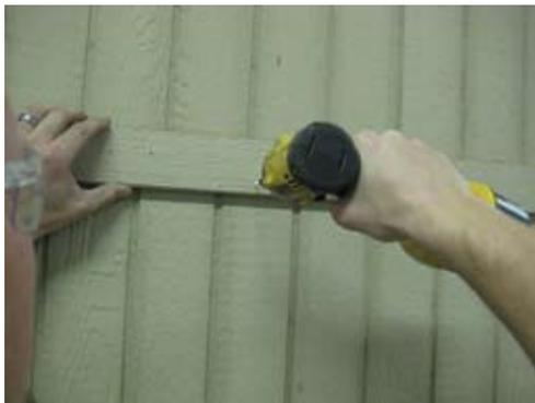
Secure gable splice trim to walls with 1 1/4" zinc screws as shown.
