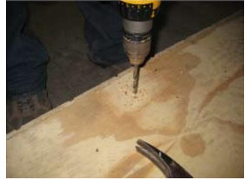
Use 3/16" drill bit and drill a hole where the barrel bolt made a mark on the floor. When closing the door, barrel bolt will insert in hole to keep door closed.
