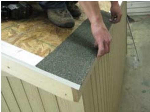
Shingles are provided by the customer. Begin by installing the starter strips as shown. Secure with 7/8" roof nails.
