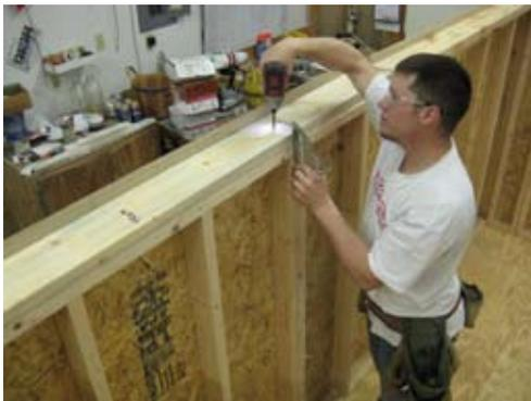
Make sure top plate is flush on inside wall.
