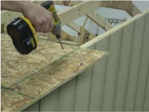
Now make sure overhang measures the same as the bottom and secure with 1 1/4" zinc screws.
