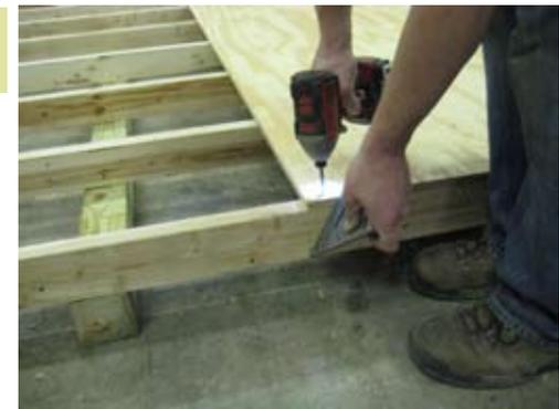
Keep plywood flush as shown and secure with 1 1/4" screws.
