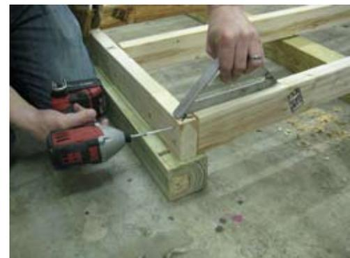
Next use square to make sure 2x4 rim is flush on top with joist and secure with 2 1/2" screw.
