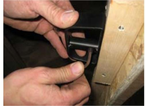
Use allen wrench to secure D-handle as shown.
