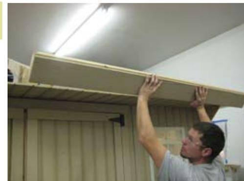
When installing fascia make sure 2x4 is up and trim overhang is down.
