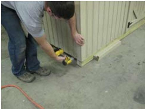
Securing corner on bottom with 1 1/4" zinc screw.
