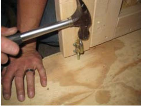
Now locate the barrel bolt located on the double door. Make sure door is closed and use hammer to tap on barrel bolt. This will leave a mark on the floor.
