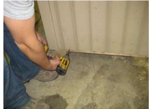
Insert 1 1/4" zinc screw every 8" to 10" on bottom edge of siding all the way around the building.
