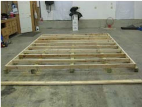
Once 4x4's are layed out, install 2x4 joist on top as shown. The 2x4's are 16" on center.
