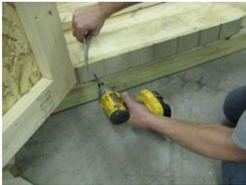
Keep flush with top of floor and secure with 1 1/4" screw.
