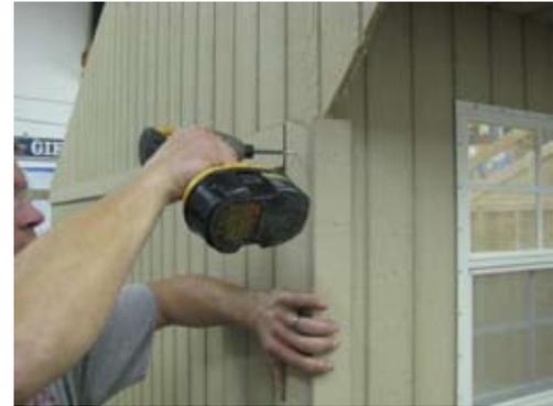
Install corner trim as shown. Secure with 1 1/4" zinc screws.
