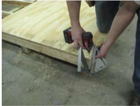
Next install 5/8" CDX flooring. Make sure plywood is flush on the outside with 2x4 as shown. Secure with 1 1/4" screws.
