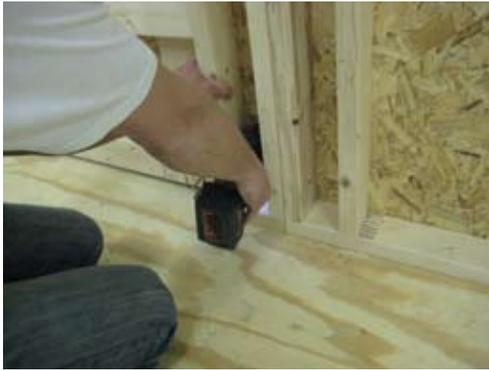
Secure walls with 2 1/2" screws as shown.
