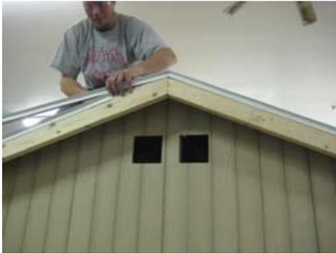
Drip edge goes around the edge of the roof as shown. You need to cut at the peak and also cut off at correct length.
