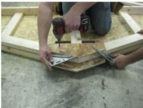
Locate OSB gussets. Install on both sides of peak. Secure with 1 1/8" zinc screws.
