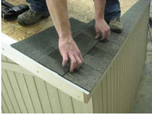
Install shingles as shown and secure with 7/8" roofing nails.
