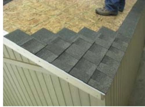
Continue installing shingles in a stepping pattern as shown.
