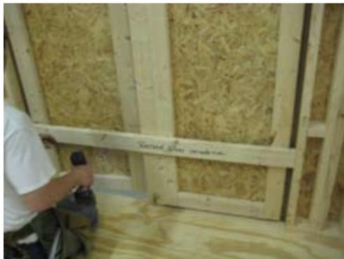
Continue with removing 2x4 from double door as shown.
