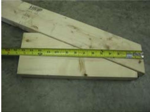
Next install heel on short end of truss. Measure 14 1/2" from truss to end of heel.
