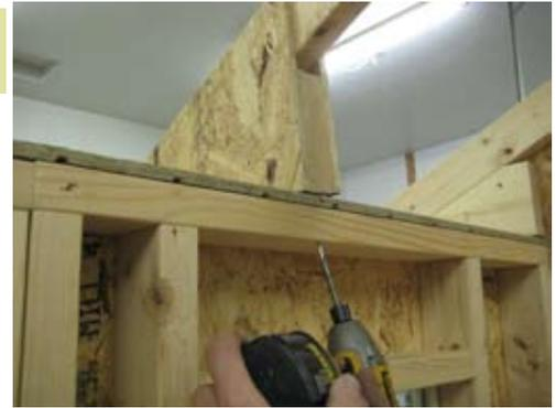
To complete truss in front secure with another 2 1/2" screw from inside as shown.
