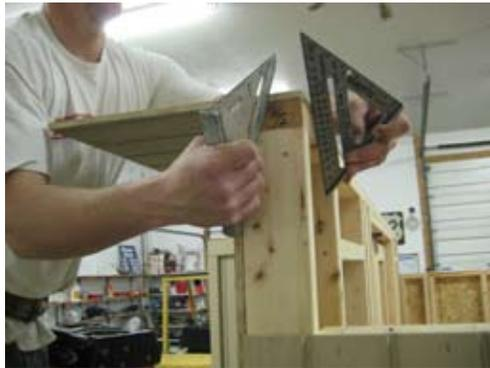
Install LP Smart siding strips on the front wall as shown. Keep flush on inside and secure with 1 1/4" zinc screws going into 2x4 top plate.
