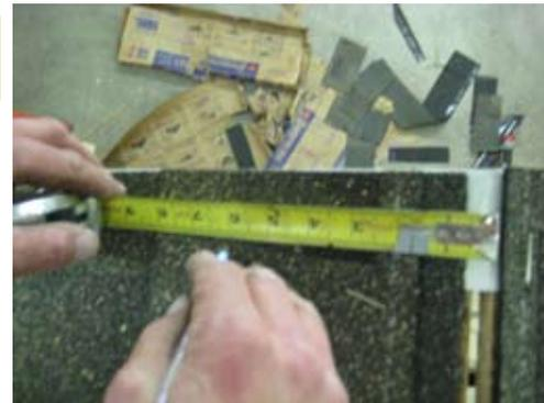
Measure 6" from the center of the peak as shown. Do this on each end at the peak.
