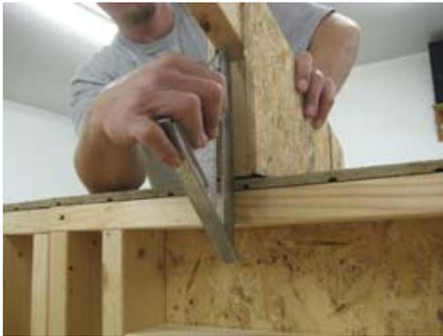
Keep heel of rafter flush on inside as shown.
